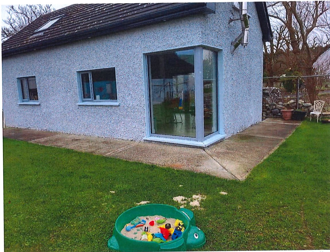
Plate 2-1 Location of the chalet with finish floor level of 4.55m OD Malin and surround ground at 4.4 to 4.5m OD Malin
